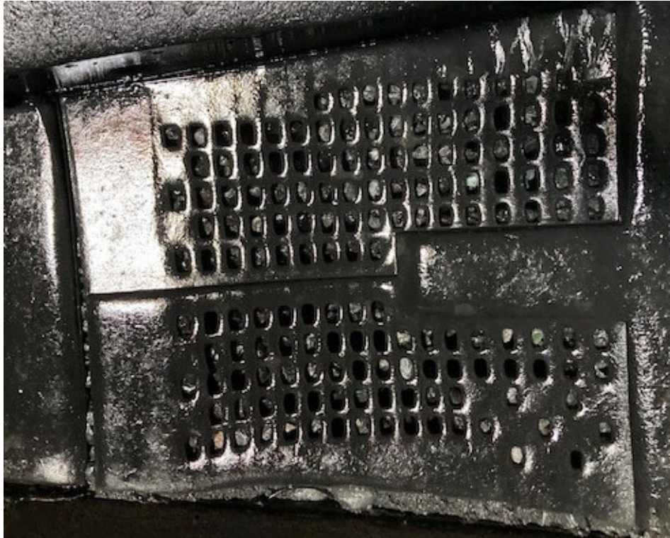
Figure 6 SAG Grate Inspections
